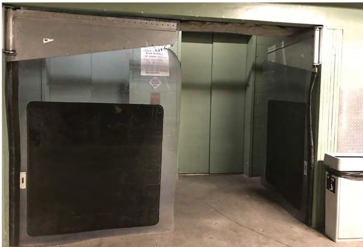
Figure 2-7. Entrance of the Freight Elevators at Seattle Municipal Tower
