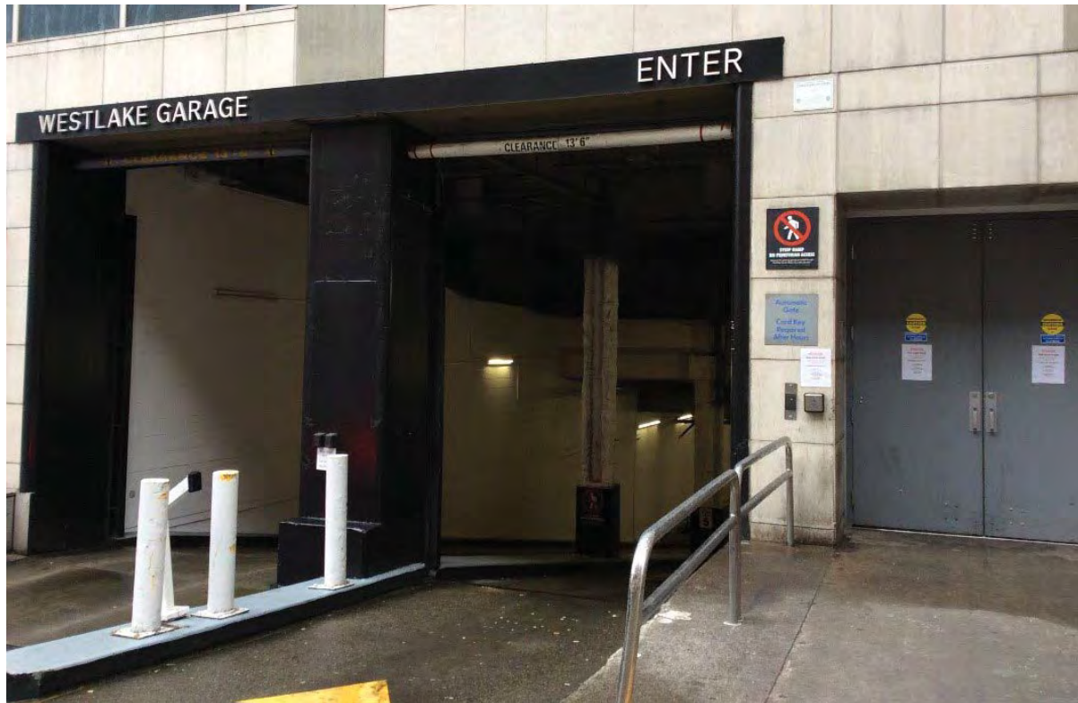
Figure 2-23. Westlake Garage on Olive Way
