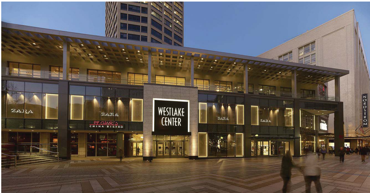
Figure 2-20. Westlake Center/Tower (Google)
