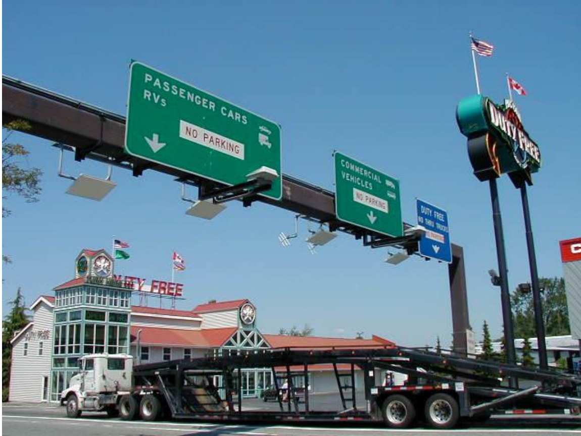
Figure 3. E-seal reader antennas on gantry at Washington-British Columbia border.
