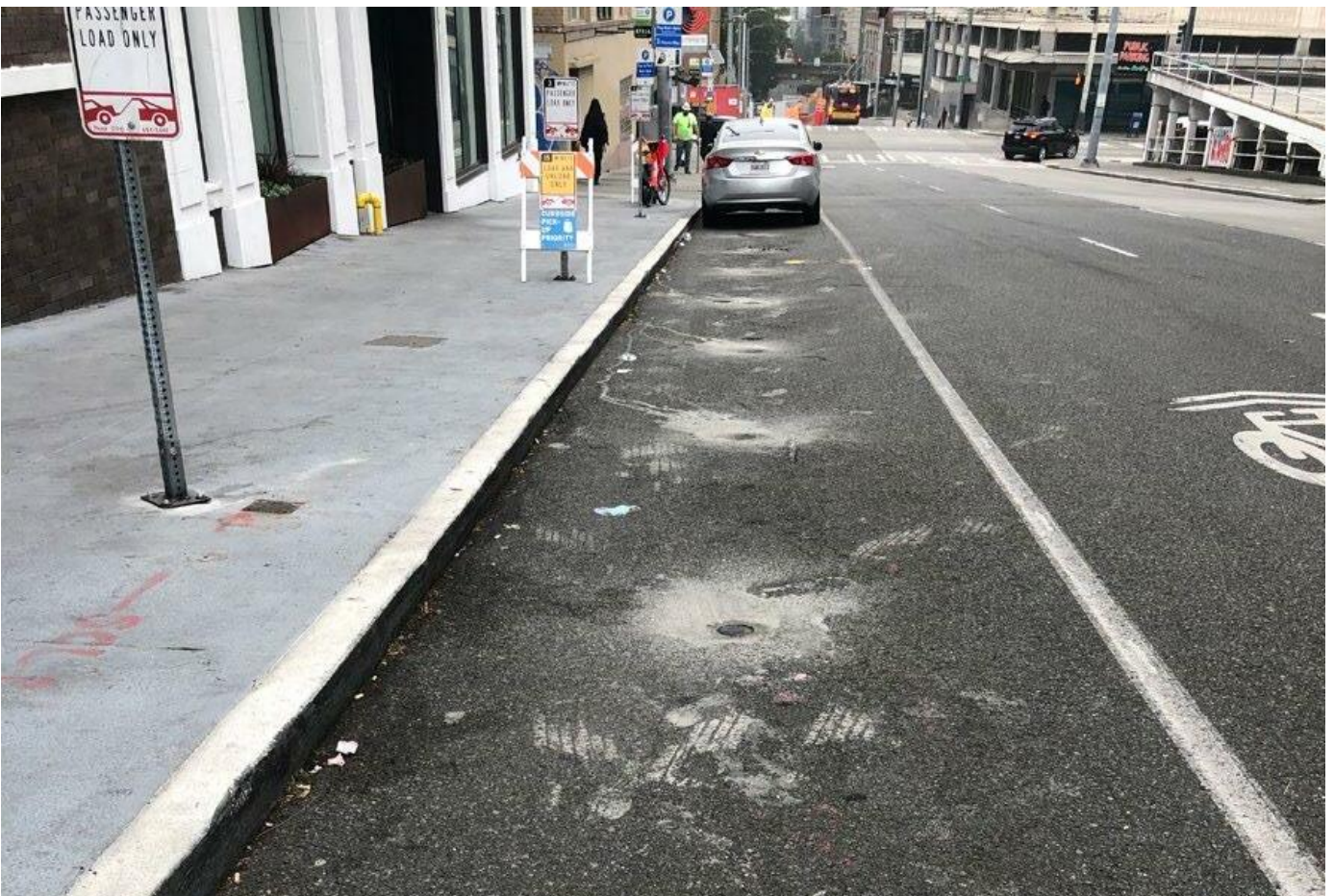
Figure 4: Deployment of curb availability sensors on a passenger load zone and commercial vehicle load zone in Seattle, WA274 curb parking availability sensors were installed on commercial vehicle load zones and passenger load zones
