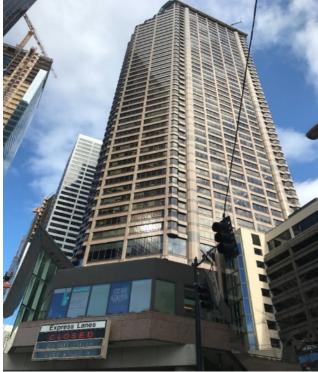
Figure 2.1 Seattle Municipal Tower
