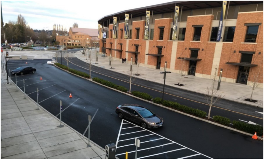
Figure 3-5. Adjacent Tyee Club Parking to UW Station
