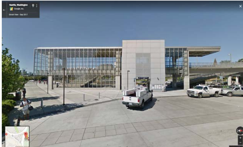
Figure 5-1. ‘Husky Train’ Proposed Site #1. UW Station on Sound Transit Right of Way (50)
