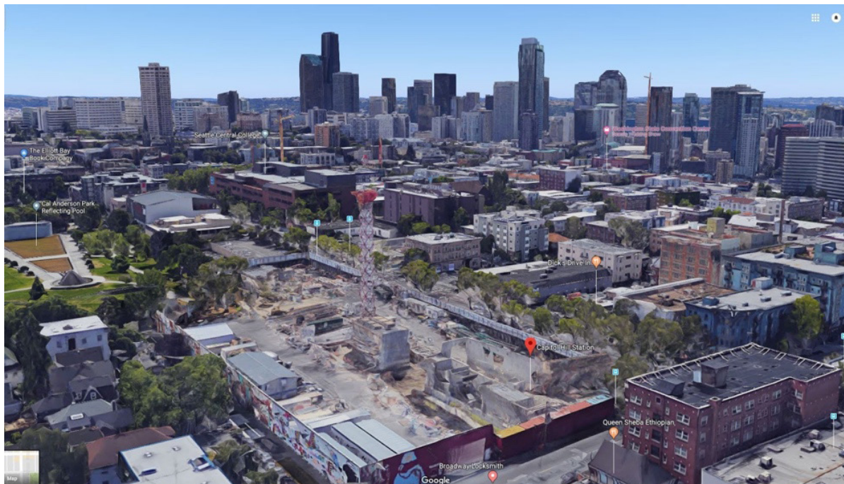
Figure 3-7. Aerial View of the Built Environment SW of the Capitol Hill Station (45)
